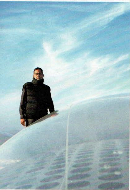
Breathing room Enric Ruiz-Geli, left, on the house's roof; its inflatable panels expand and contract to let in and block out light. Opposite: the house, photographed under construction, is conceived as a series of spaces grouped around an elevated courtyard pool.
